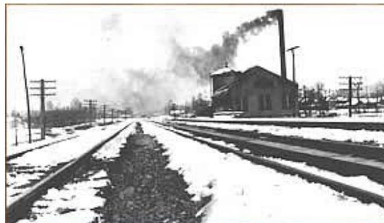
Thawing effect of buried heating pipes is seen at Bellwood Pans.
