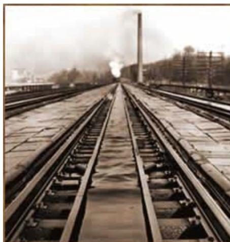
As a New York Central train approaches the New Hamburg Track Pans, turbulence in the pan is created by the onrush of water from the filling inlets on the sides. Note the concrete slabs to curtail erosion, the ever-present heating/pump plant, and the heating pipes protected under metal curbing adjacent to tracks.
