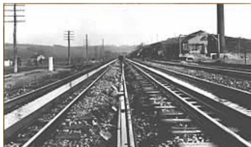
Wilmore Track Pans, October 1906. Laying heating pipes in trench between tracks.
